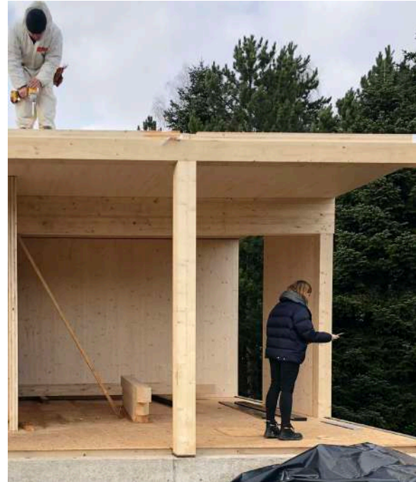
image 5: upgrading a 1970's concrete building with a wood construction, 2001.
