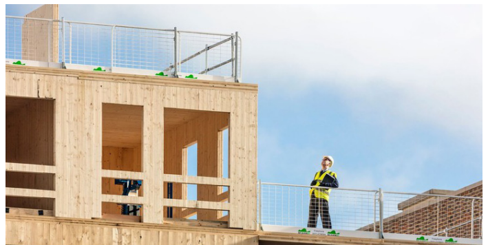
image 15: World's Largest CLT Building Provides a Model for High Density Urban Housing (2018) [photograph]. https://www.archdaily.com/903839worlds-largest-clt-building-provides-a-model-for-high-density-urban-housing
